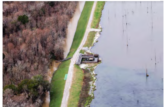
Figure 19. High-water event on February 3, 2016 with water levels approaching dam sides.
