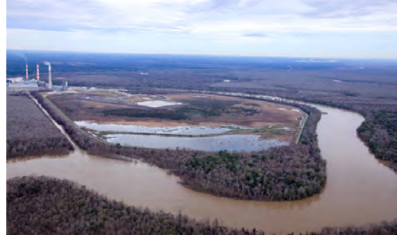
Figure 18. Aerial showing a high water event at Plant Barry.
