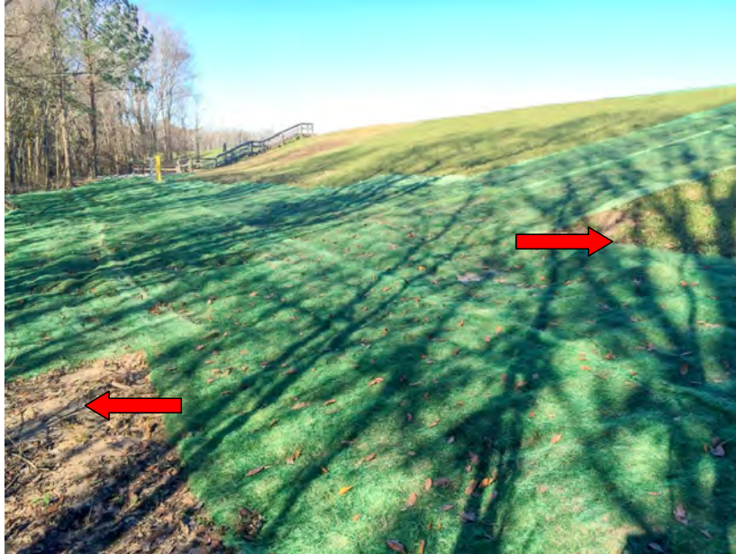
Photo 2: Evidence of Piping North of Pond Outlet (Feb. 4, 2016)
