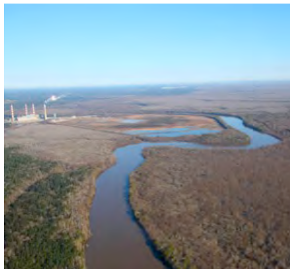
Figure 8. Aerial of the Mobile River wrapping around the coal ash pond at Plant Barry.
